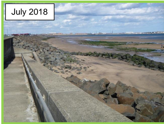
Little Scar access ramp in 2018 (/C0401C33)
