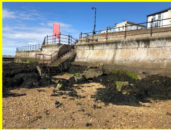
Low beach levels at access steps (/C0401C04)
