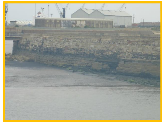
South face of North Pier (C0401C22)
