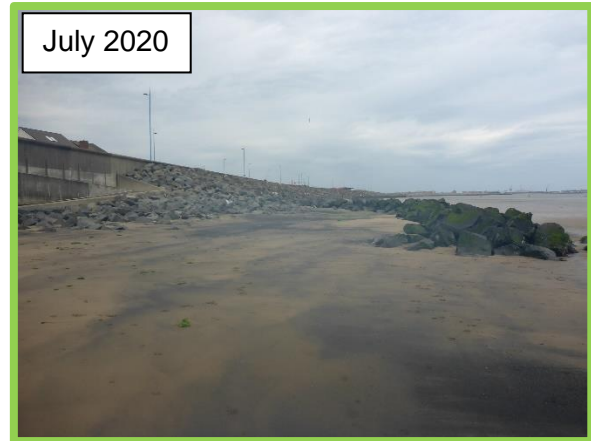
Little Scar access ramp in 2020 (/C0401C33)
