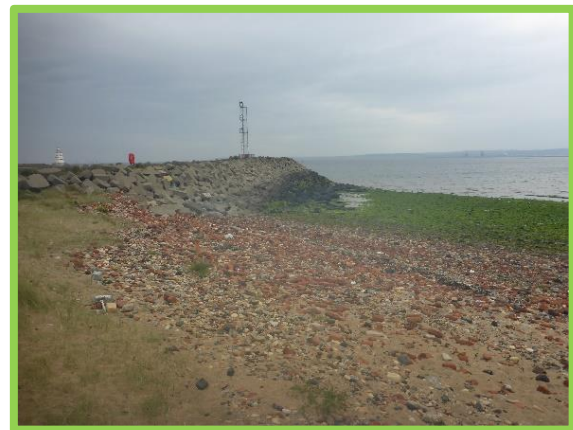
Middleton Jetty south aspect. Buildup of construction rubble in the foreground (/C0401C16)
