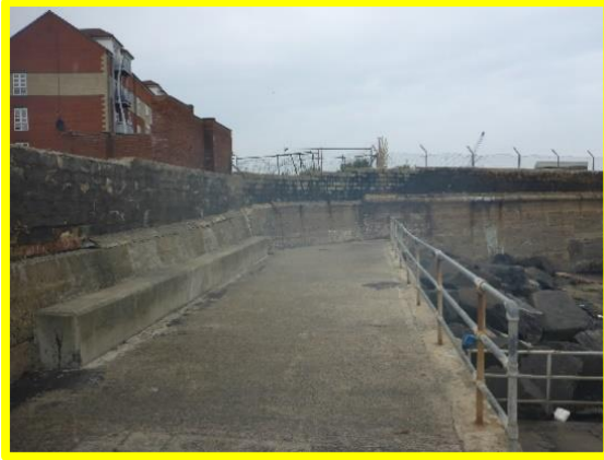
Access structure to Middleton beach in fair condition (C0401C20)
