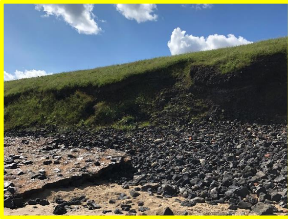
Recent local slope failure (/C0302C03)
