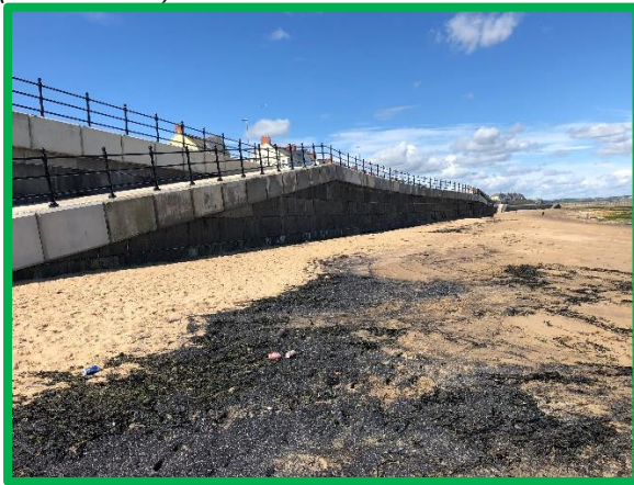
As built condition access ramp at Arabella Street, previously undercut (/C0303C01)
