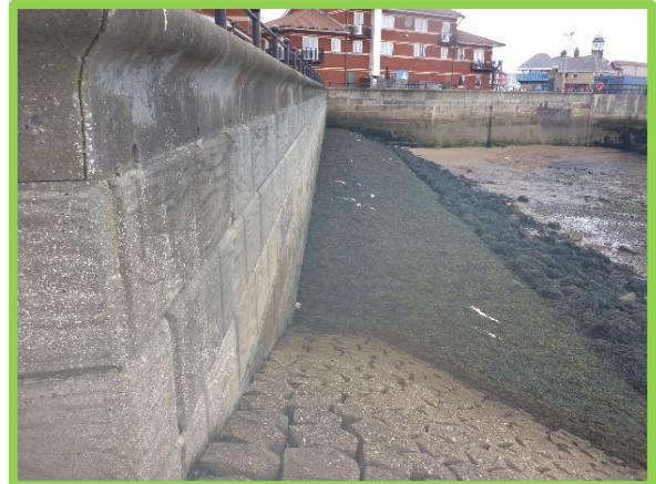
Concrete blockwork revetment obscured by vegetation (C0401C25)
