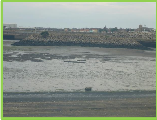
Rock revetment breakwater in good condition bar mature vegetation growth (/C0401C30)
