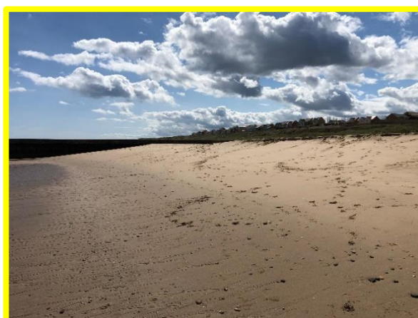
Piled outfall structure retaining sediment on its north side. (/C0302C01)
