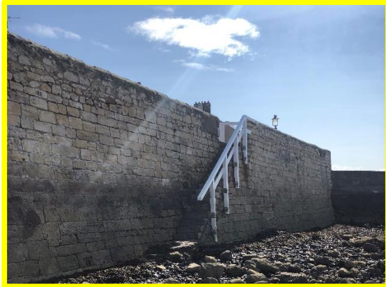
Repaired handrailing and beach access steps (/C0401C35)
