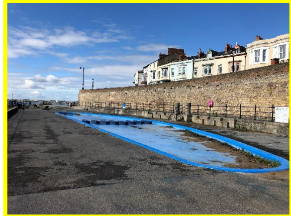
Rear masonry wall in fair condition (/C0401C04)
