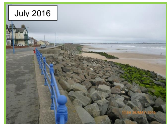
Little Scar access ramp in 2016 (/C0401C33)
