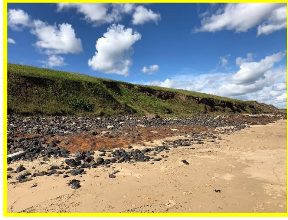
Historic large slope failure (/C0302C03)
