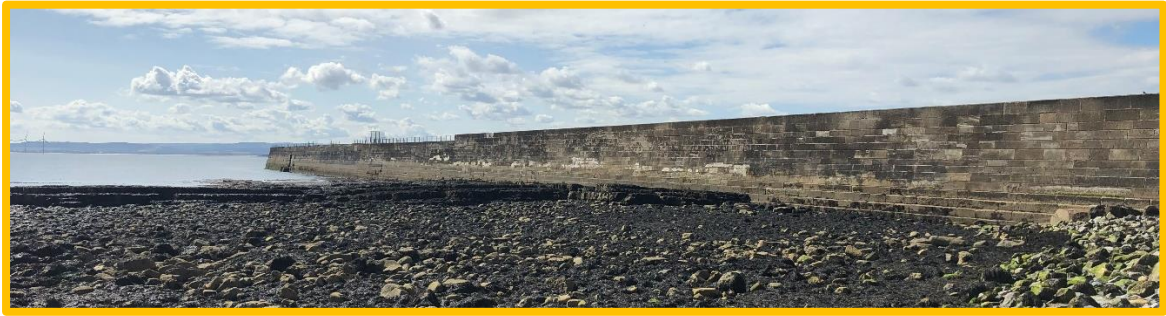
Heugh Breakwater – landward end north aspect (/C0401C01)
