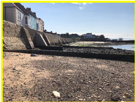
Recently constructed outfall and abutment. (/C0401C35)
