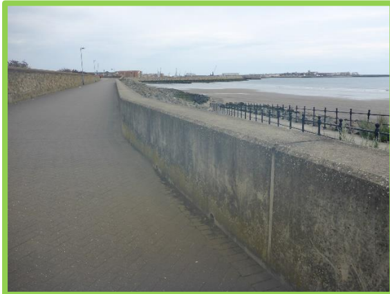
Concrete sea wall and repaired slipway handrail (/C0401C33)
