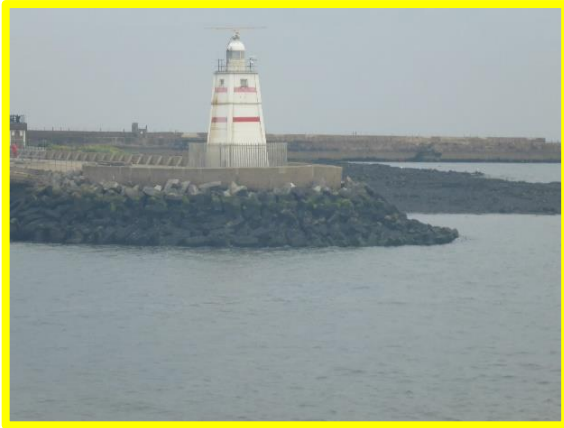
Accropode armour units around pier head taken from Middleton Jetty (/C0401C34)
