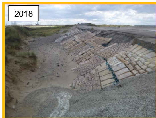
South face of North Gare Breakwater. Dune field in lee of structure (/C0503C01)
