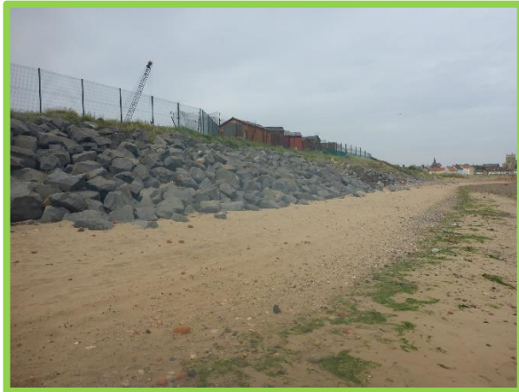
Rock armour revetment and Gabion wall looking towards Middleton Jetty (/C0401C17)
