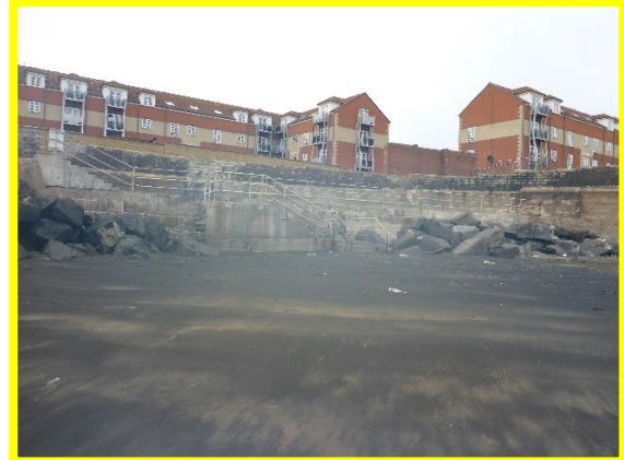
Access structure to Middleton beach in fair condition (C0401C20)
