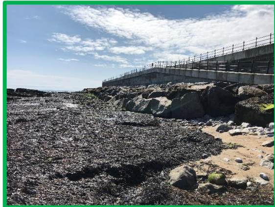
As built condition sea wall – inaccessible foreshore to the south. (/C0303C02)
