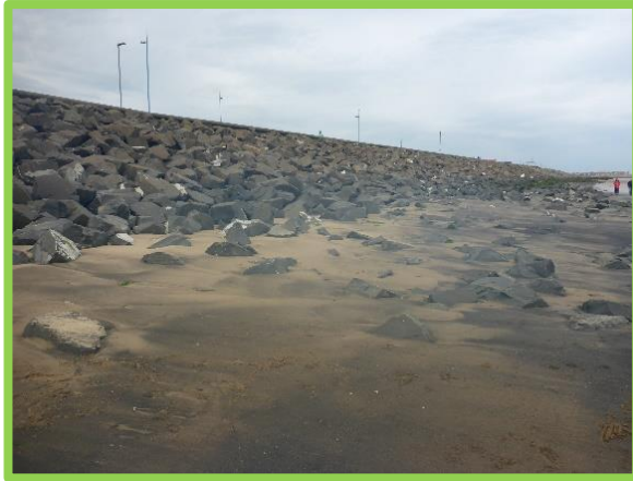
Rock armour revetment and concrete seawall (/C0401C33)
