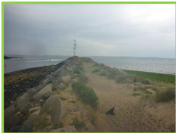
Middleton Jetty north aspect (/C0401C16)
