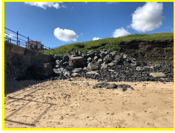
Rock armour revetment at Marine Drive seawall (/C0302C03)
