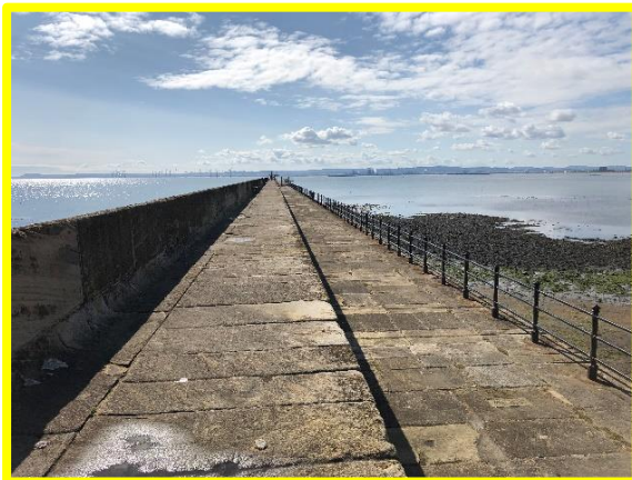
Heugh Breakwater – Deck slab (/C0401C01)
