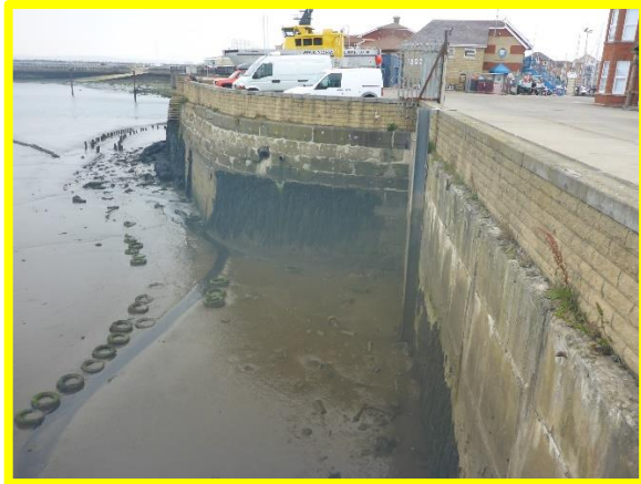
Local repairs to masonry seawall to north of harbour entrance (C0401C24)
