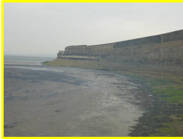
North face of North Pier (C0401C22)
