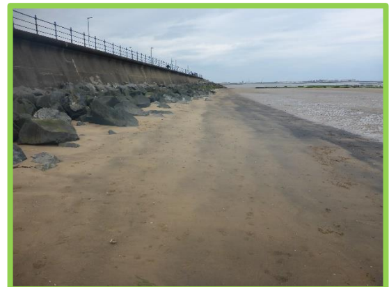
View looking north. High beach levels concealing toe of revetment structure. (/C0501C05)
