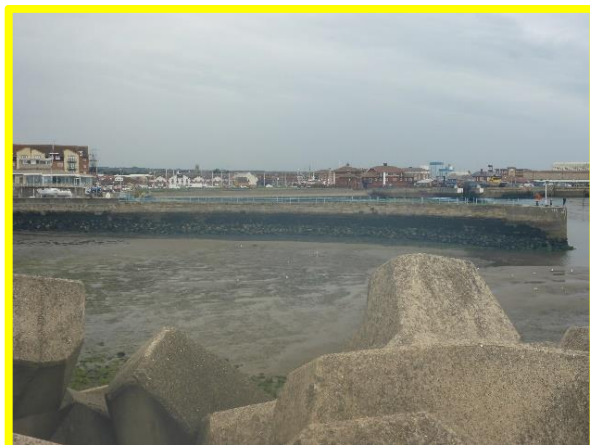
Outer face of Middle Pier (/C0401C28)
