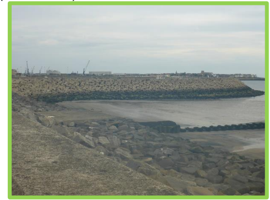
Outer face of South Pier (/C0401C32)
